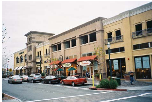
Parking Structure with Ground Floor Retail in Walnut Creek
