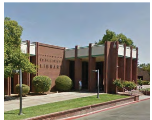
Yuba County Library on 2 nd Street
