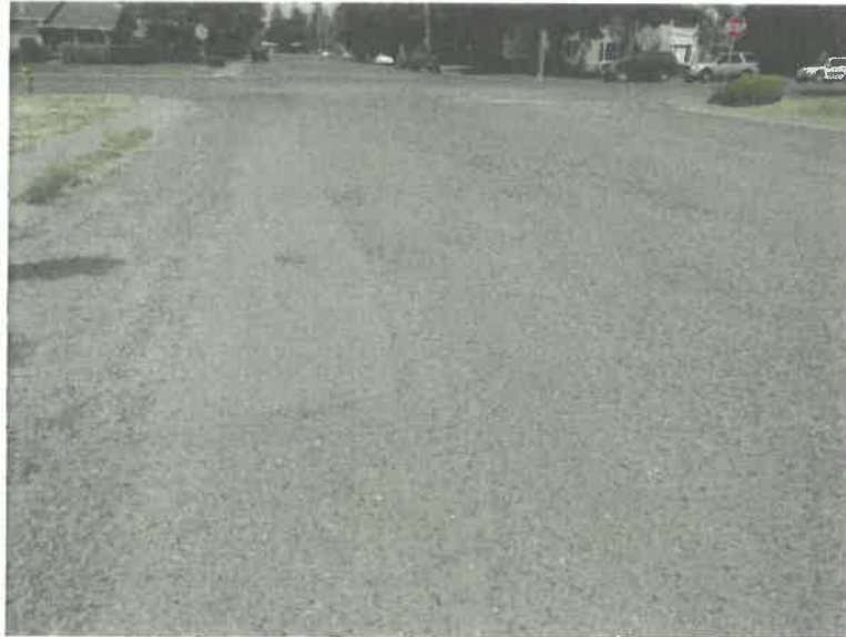
Example of: High severity raveling - Sweezy St between 16 th St and 17 th St (PCI 8)
