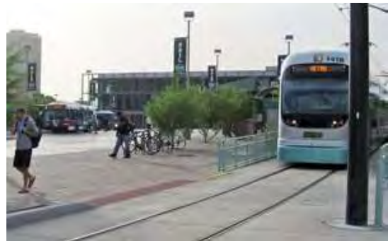
Tempe, Arizona's Transportation Center is light rail and bus hub with bicycle storage and repair facilities.
