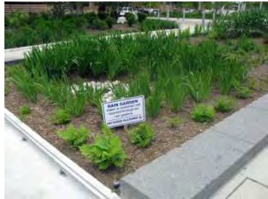
This rain garden in Washington, D.C., captures and reuses stormwater.
